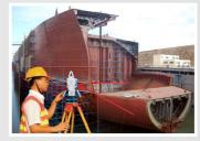
Large shipbuilding surveying and positioning
